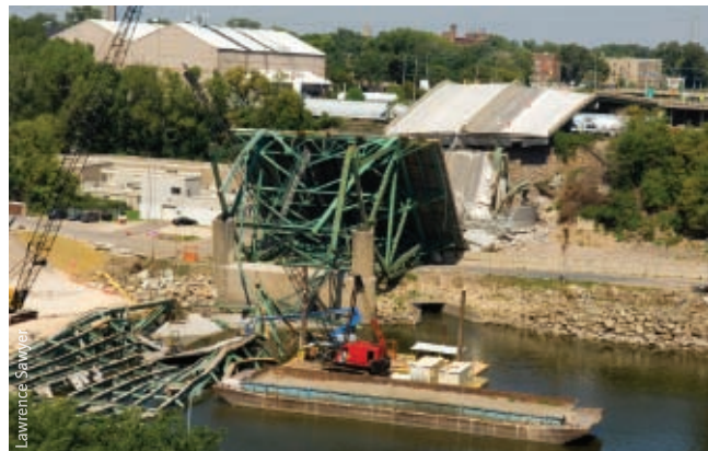
I-35W in Minneapolis collapsed partly as a result of a bridge inspector not realising the significance of buckled gusset plates
