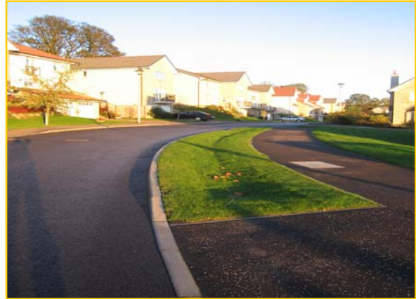
Swale drainage, Dundee
