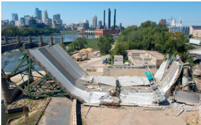
I35-W Bridge collapse in the US highlighted the need for more rigorous inspection
